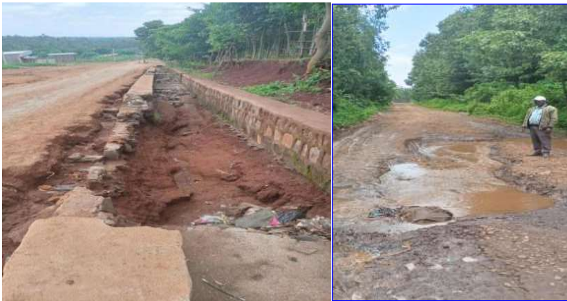
Fig.4: Road condition survey of Boditi to Badessa
