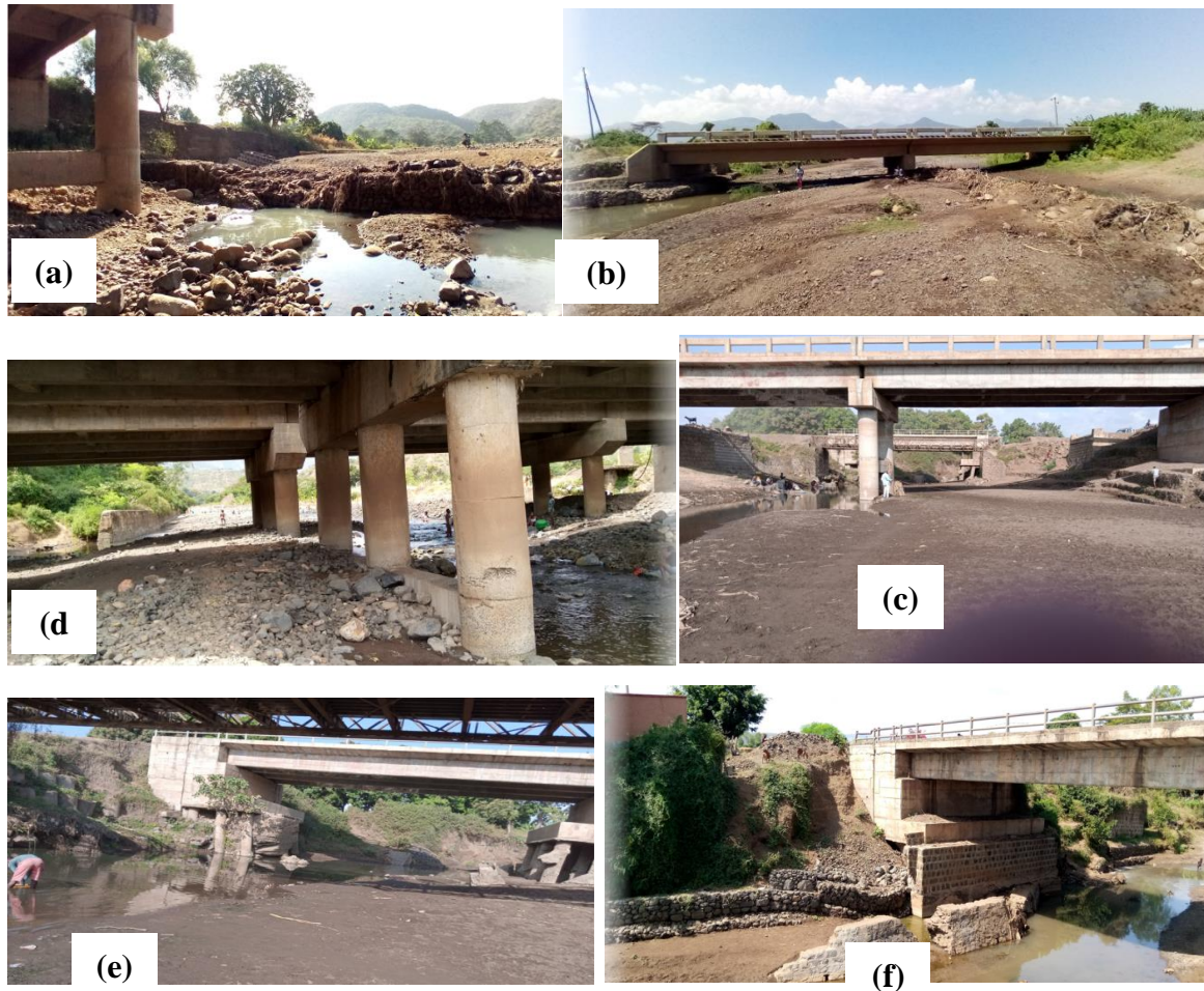
Figure 3. Scour susceptible bridges site photos
