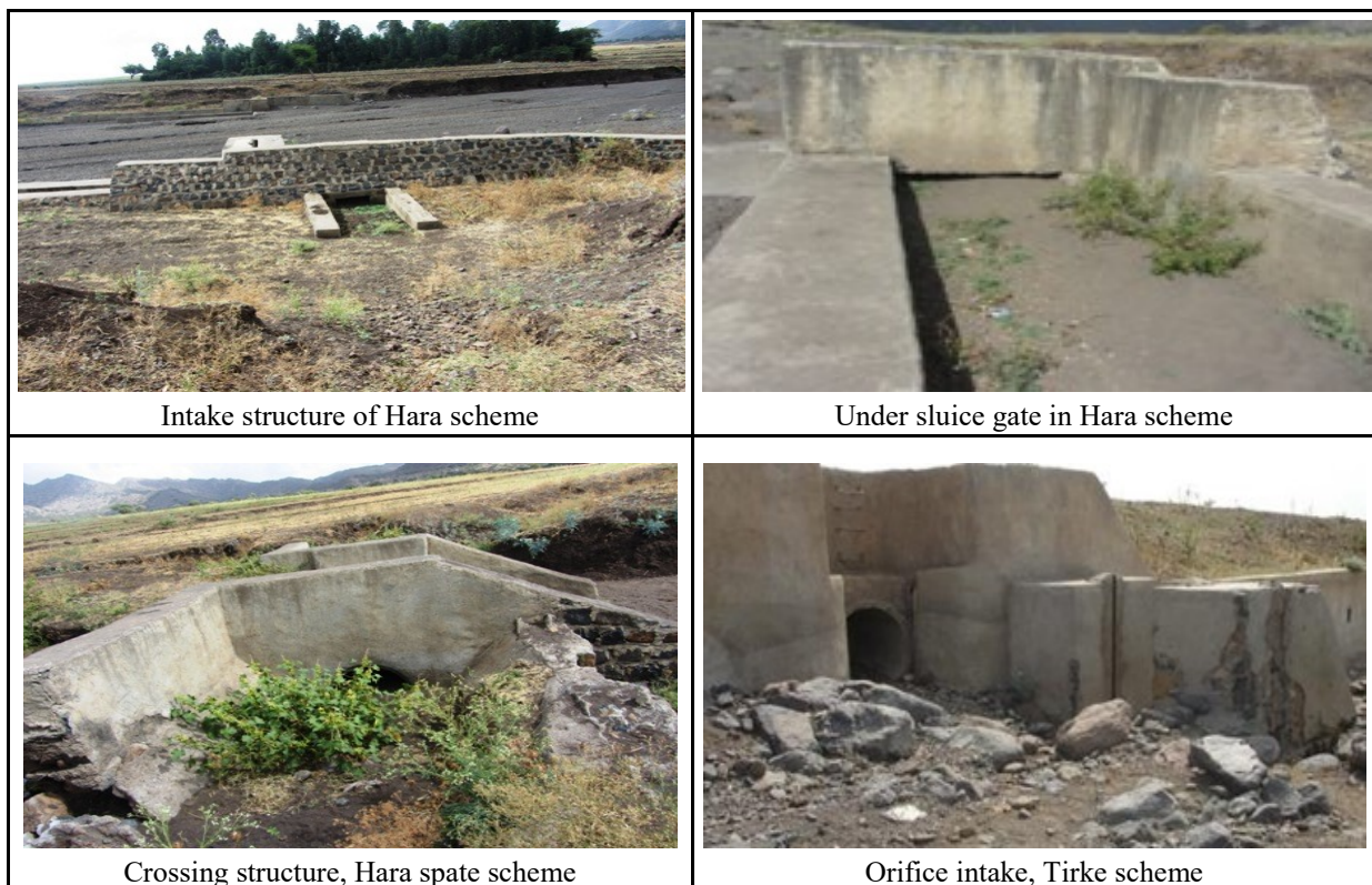
Figure 2. Headwork structures of Hara and Tirke schemes
