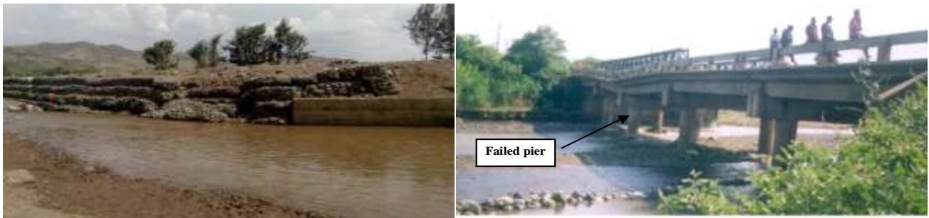
Figure 20: Kulfo flooding problems: Failure of Gabion upstream of New bridge (Left); Photograph of Kulfo Bridge after its failure during the October 1997 flood (Right)
